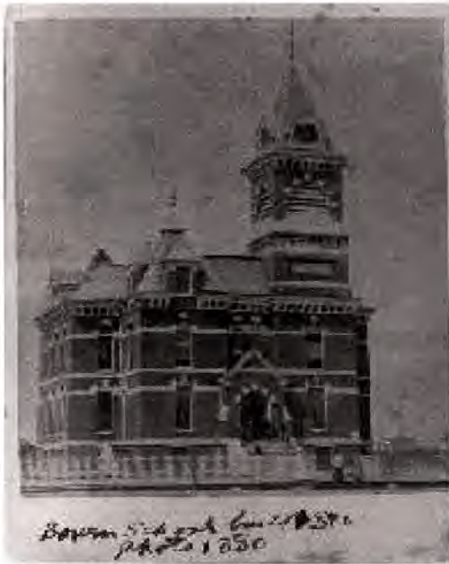
Original Bowen School located at 93rd and Houston, built 1876
